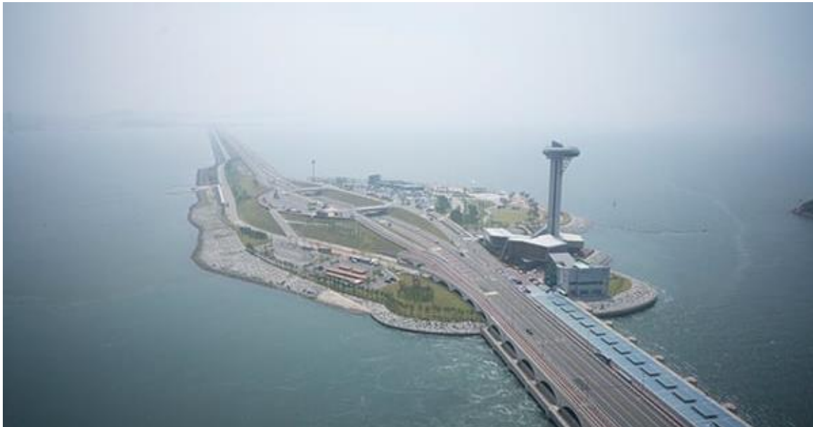
Figure 6: Lake Sihwa Tidal Barrage Power Plant
