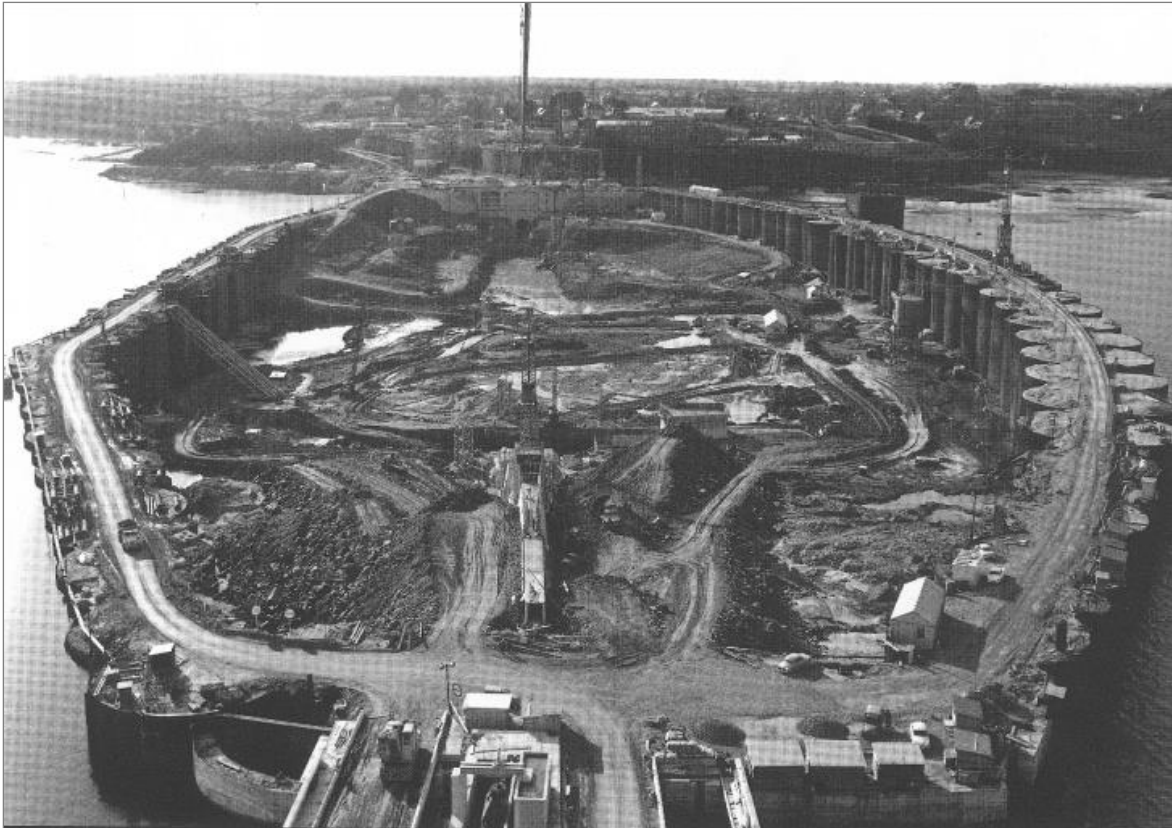
Figure 5: Main barrage cofferdam for La Rance
