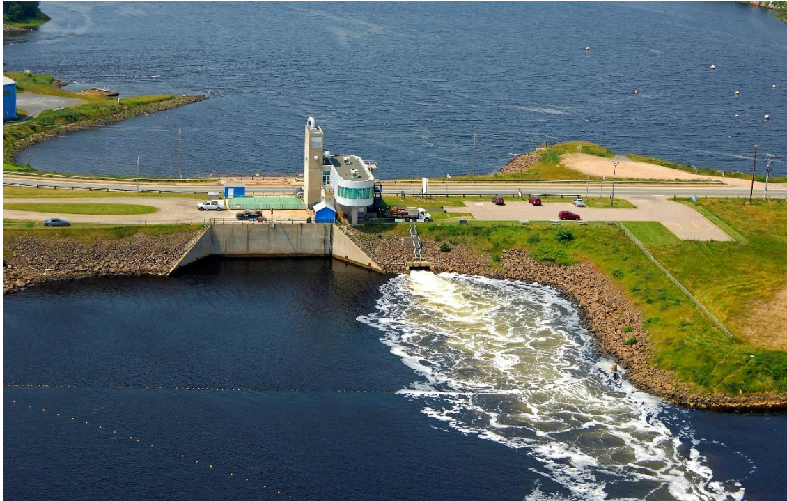
Figure 8: Annapolis Royal Tidal Station
