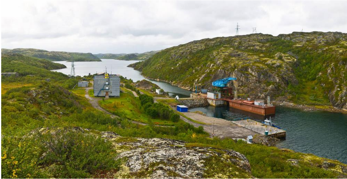
Figure 10: Kislogubskaya Tidal Power Plant, Murmansk, Russia
